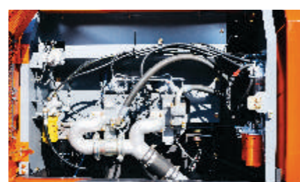
Grouped remote filters and inspection points
